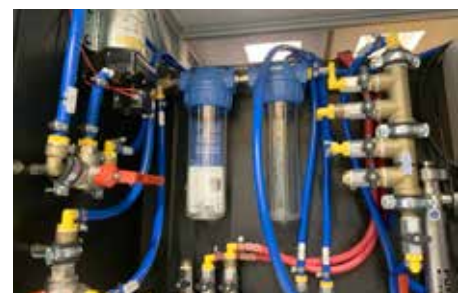
Installation of the water system.
