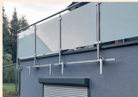
A continuous MiniTec profile replaces delivered fastenings that are too short.
