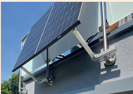
A continuous MiniTec profile replaces delivered fastenings that are too short.
